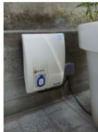
Home installation – France
