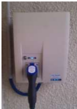
Home installation – France
