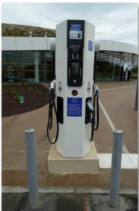
FR : La Chaponne Service – A6 Highway
